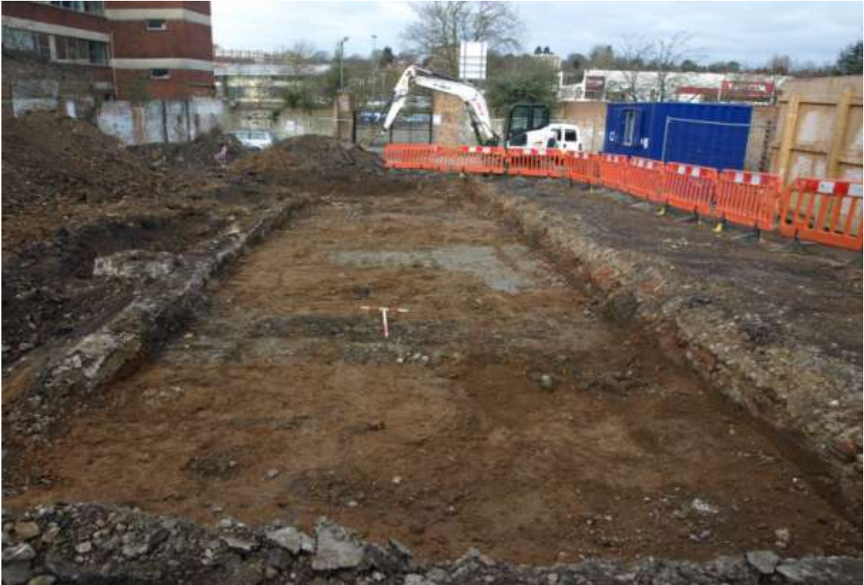
Plate 5. Showing exposed Area 2 comprising the northern part of the site, the linear formation 24 visible to the left. Looking west one and half-metre scales.
