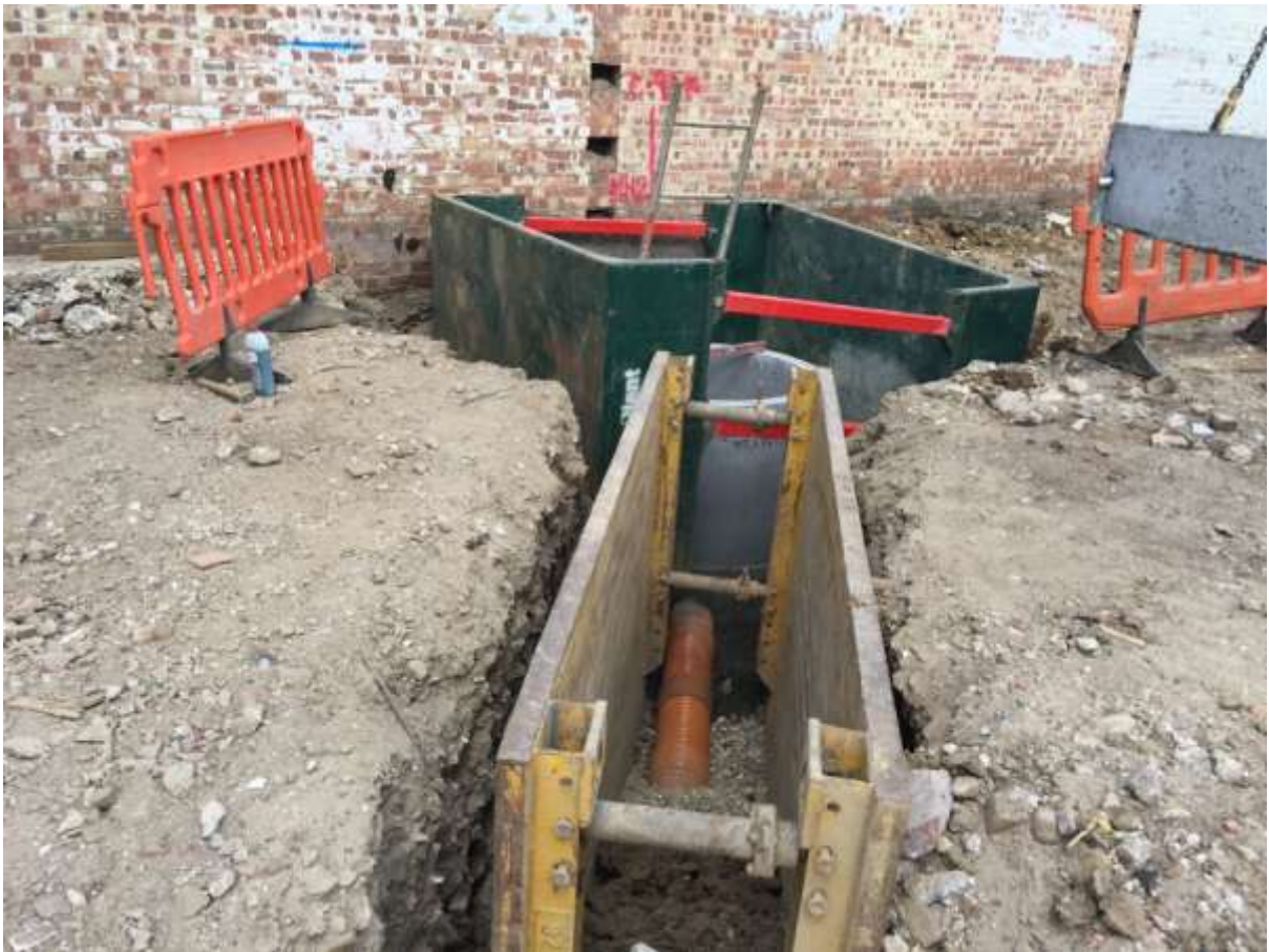
Plate 2. Drainage being installed (in made up ground)
