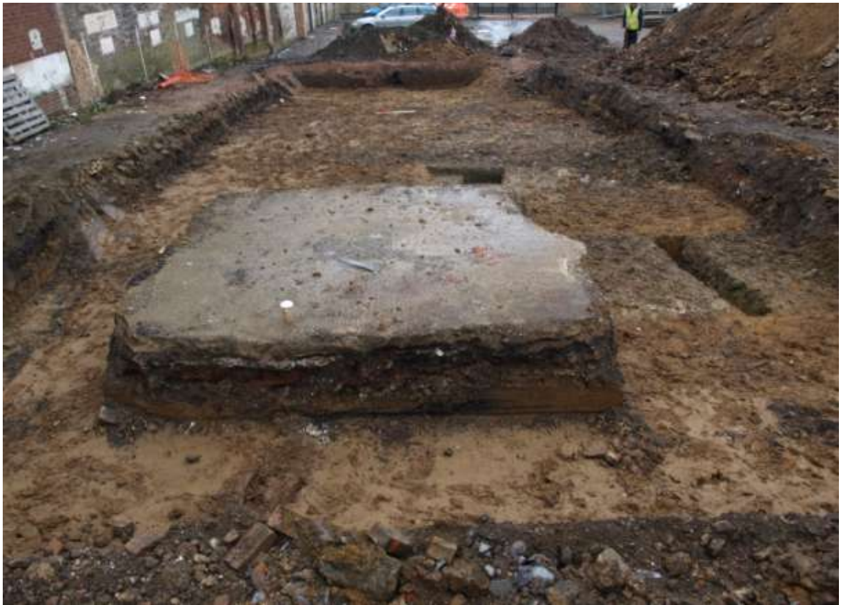
Plate 1. Showing exposed part of the site, the well feature visible in foreground. One metre scale in background, looking west.
