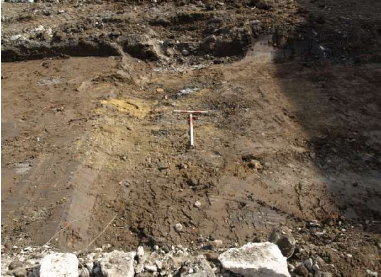
Plate 11. Showing the ground beneath the concrete footings (after they've been removed). Looking east, one and half metre scales.
