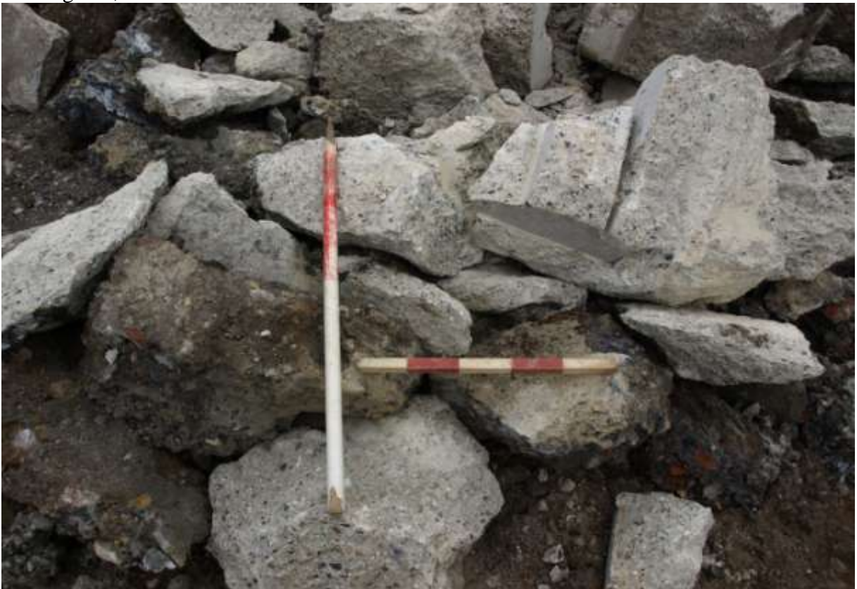
Plate 12. Showing the details of removed concrete footings. One and half metre scales.
