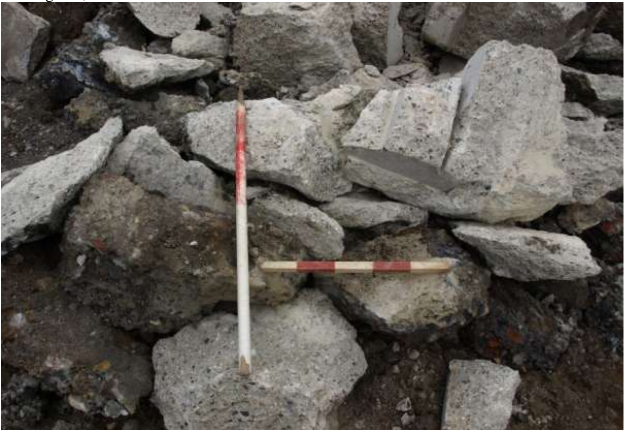
Plate 12. Showing the details of removed concrete footings. One and half metre scales.
